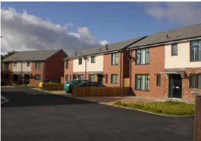
Above: Affordable housing units on Portree Road, Blackpool completed in January 2011.
